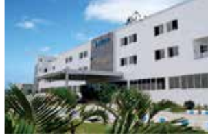
Rudrapur Plant (Green Building)
